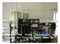
A powerful and versatile technology in removal of dissolved impurities, it finds great use in drinking water applications, desalination of sea water and for process applications. Often ground water is found to be so hard that the only way to soften is to treat it through RO and make is suitable for cooling tower make up.
